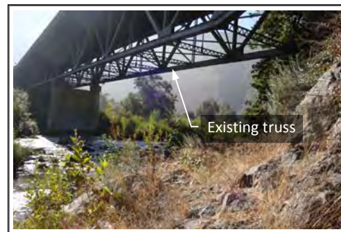
Alt 4: Hang pedestrian crossing on existing truss
