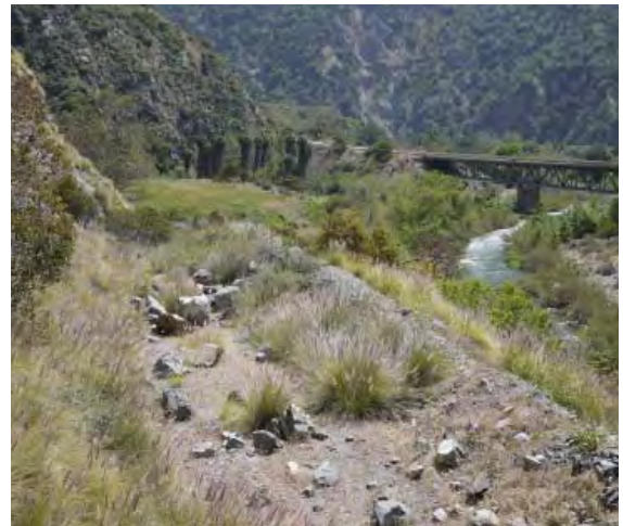
Fig. 5-2 The old road cut on the Western Bank hillside
