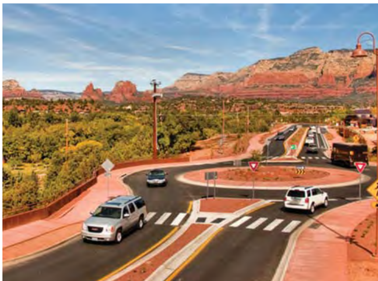
Fig. 4-2 An example of a roundabout and crosswalk
