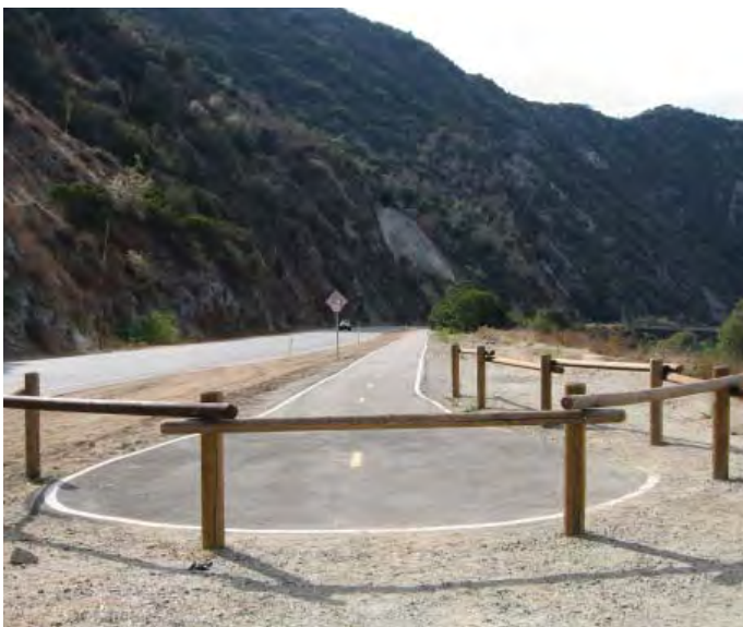
Fig. 4.1, End of the existing Class I bicycle path on Highway 39
