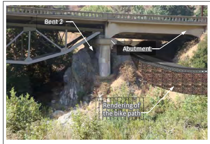
Alt 2: Bike path between the abutment and Bent 2
